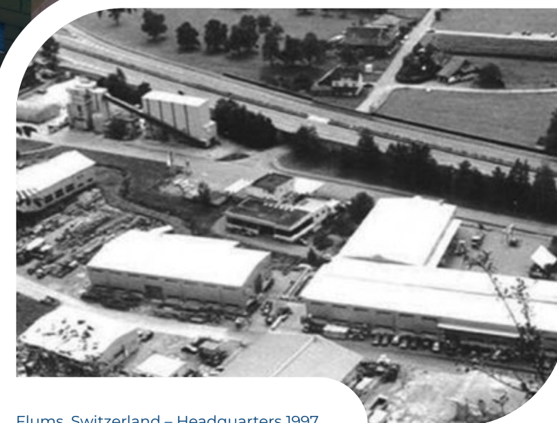
Flums, Switzerland – Headquarters 1997
