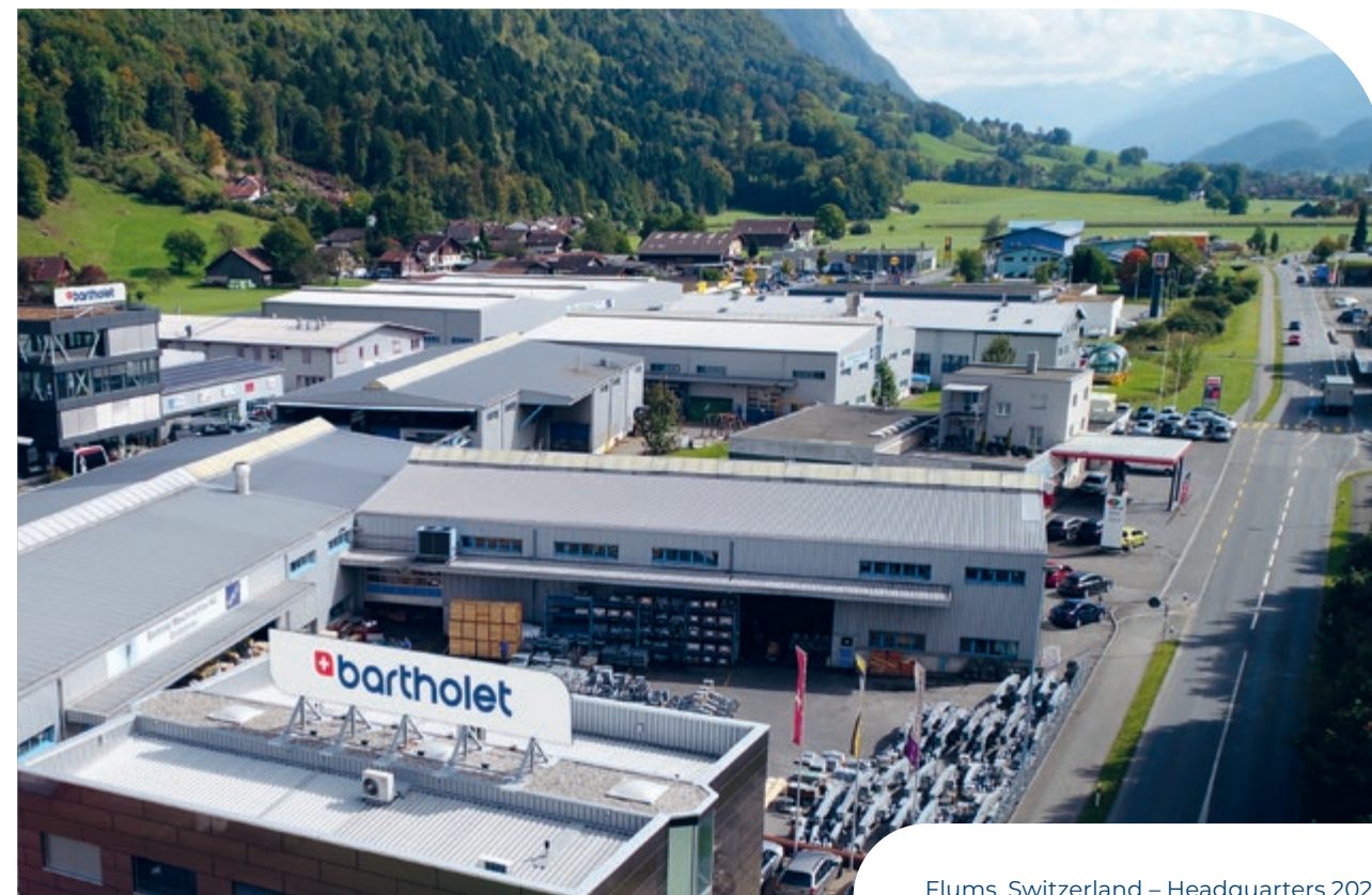
Flums, Switzerland – Headquarters 2025
